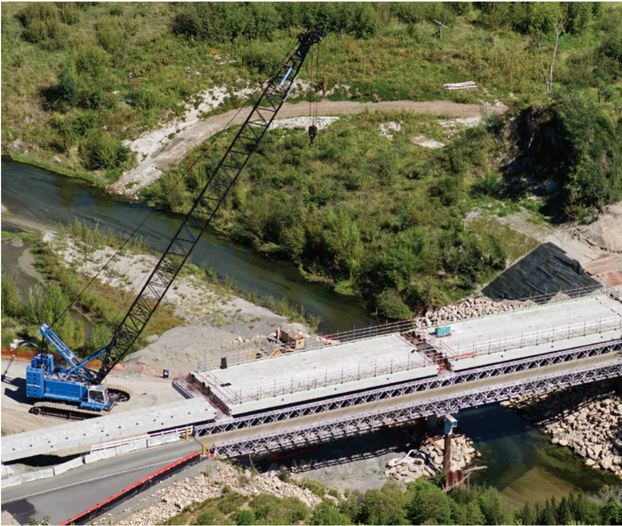
Rissington Bridge, Hastings District Council - Cyclone Recovery
