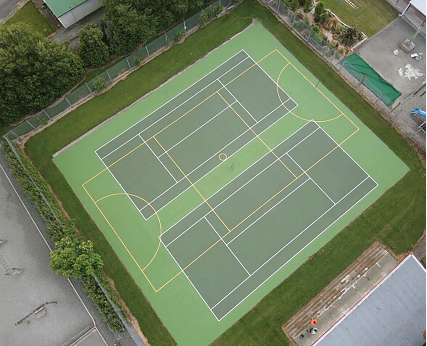
Mossburn Tennis Court Resurface - Mossburn, Southland
