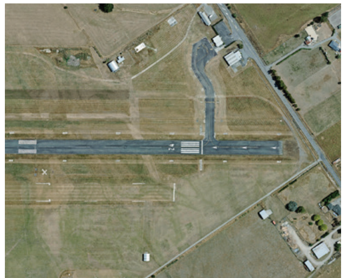
Hood Aerodrome infrastructure upgrade
