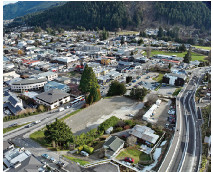
Queenstown Arterials - Stage 1
