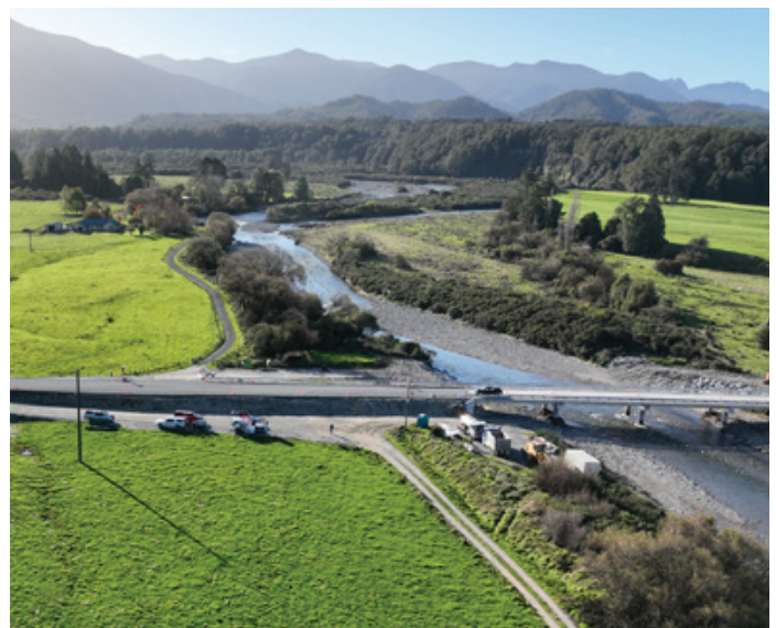
Moonlight Creek bridge replacement
