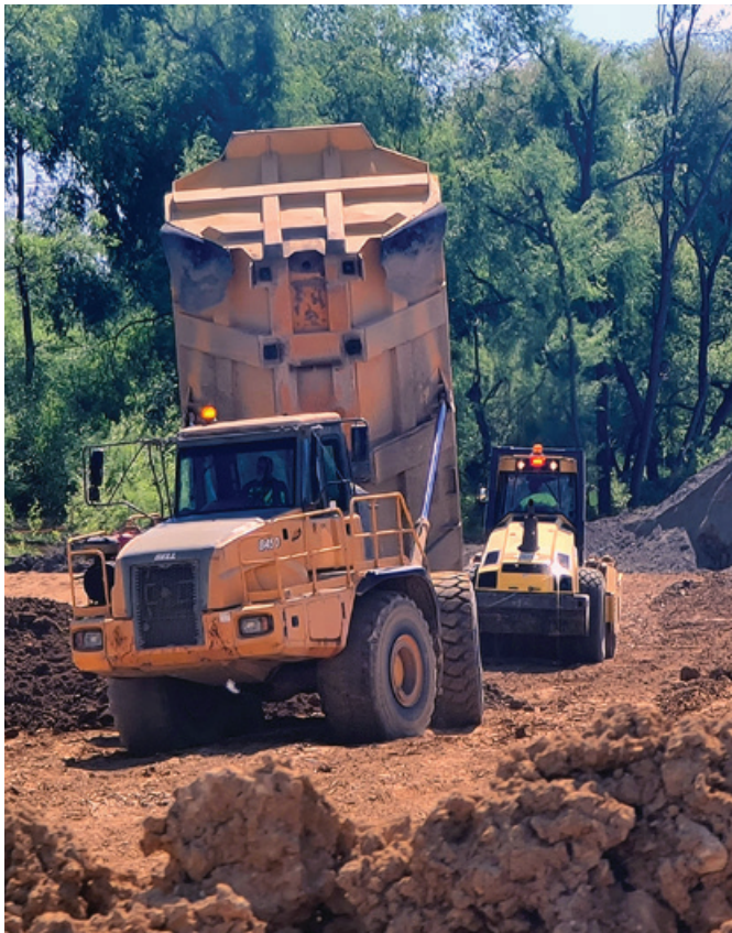
Waiohiki Stopbank Construction
