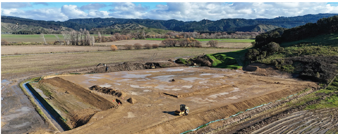
Hinemaurea Marae Rebuild, Gisborne
