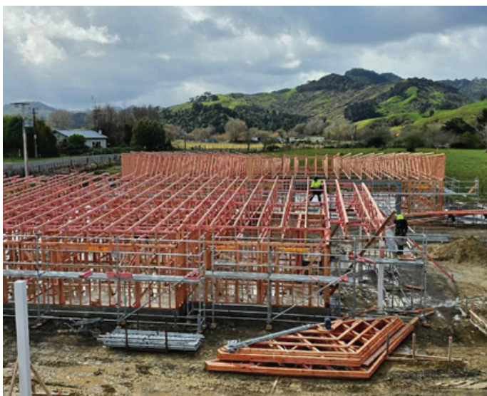
Rangatira Marae Rebuild, Gisborne
