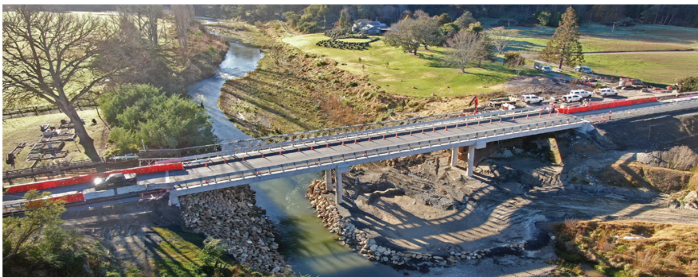
Pekapeka Rissington Bridge, Hawke's Bay
