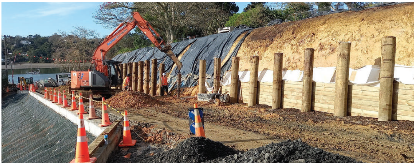
Auckland Council – Twin Wharf Road
