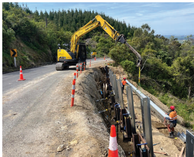
Hastings District Council – Taihape Road Slip Repairs
