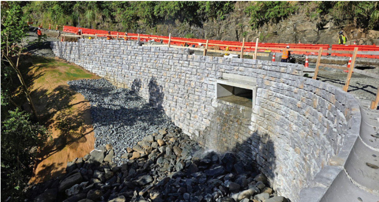
Matakana Valley Road Culvert, Auckland – Cyclone Recovery
