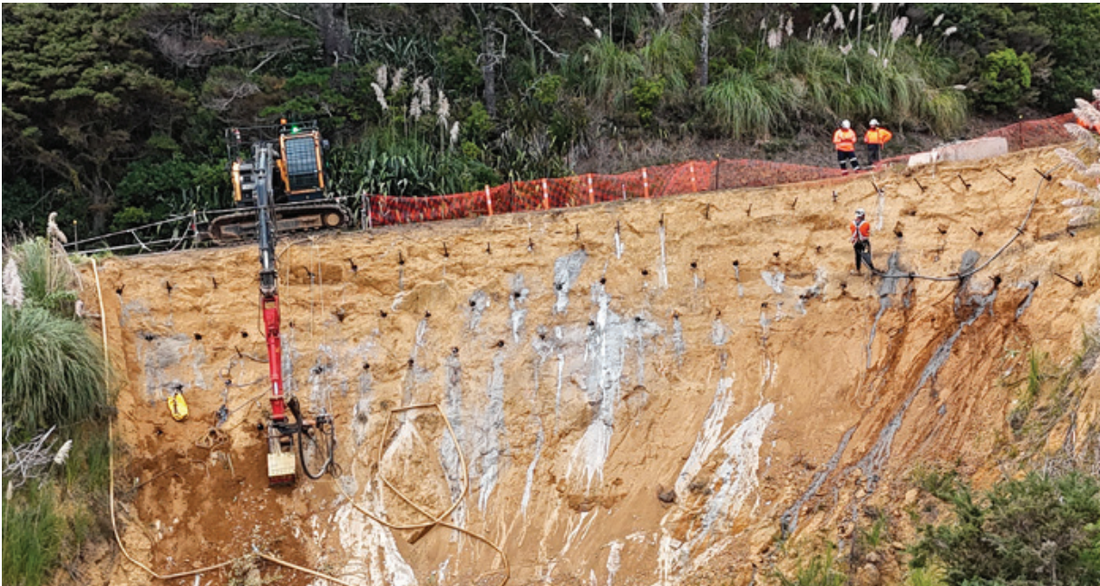
Kemp Road Slip, West Auckland – Cyclone Recovery
