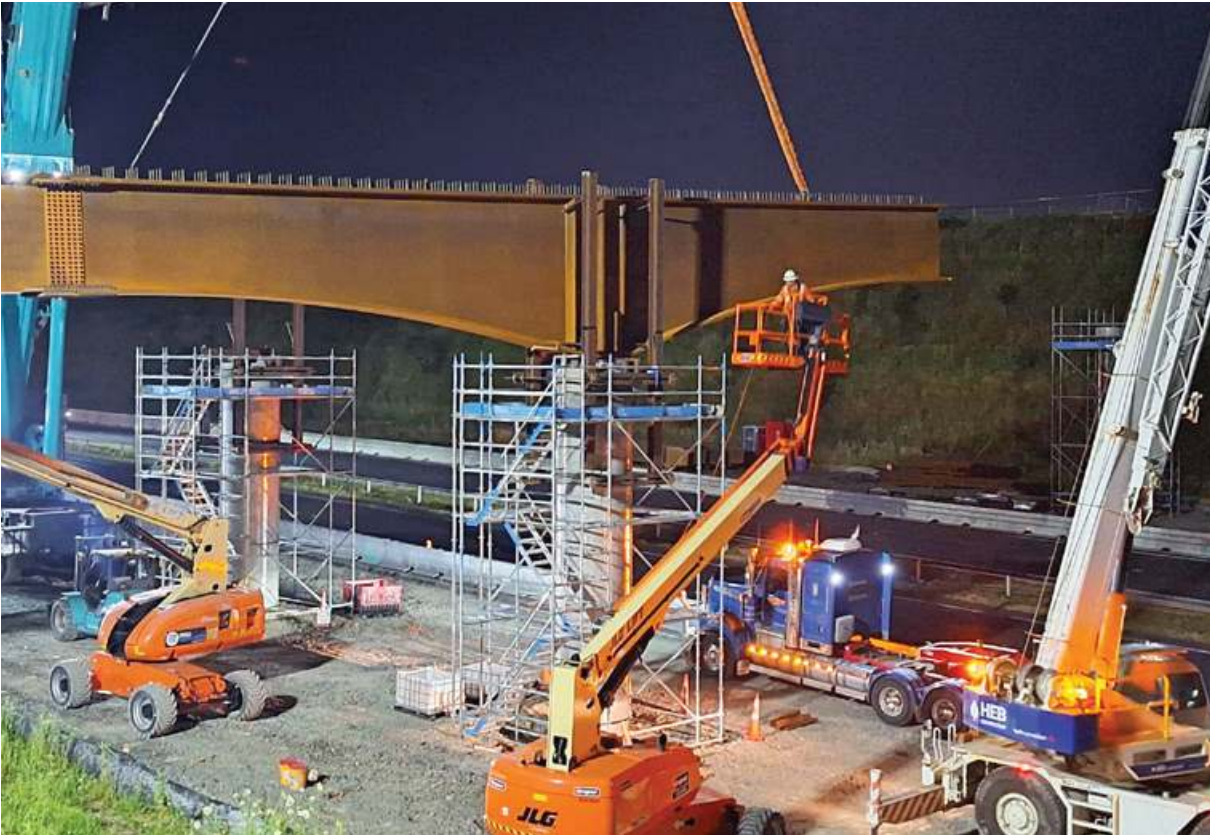
Highgate Bridge, Milldale, Auckland - IFF Programme
