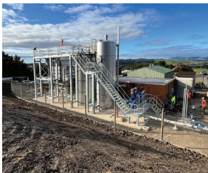
Kaihoko Combined Developments - Water Treatment Plant
