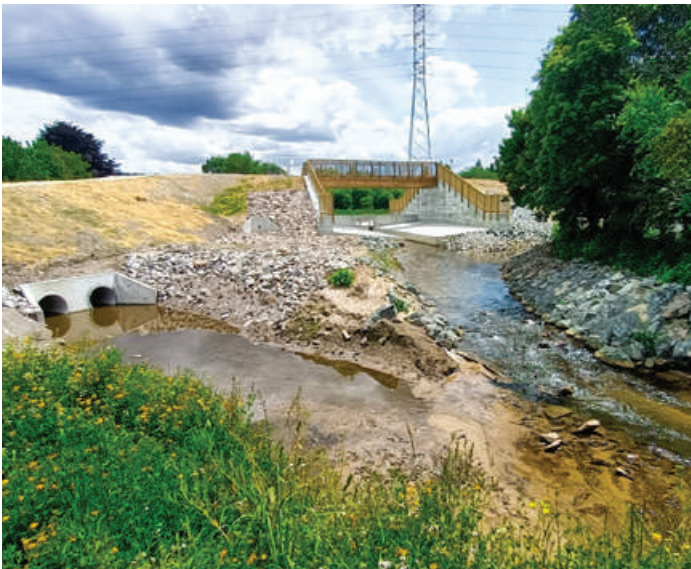
Central & Western Area Development - Linton Park Dam
