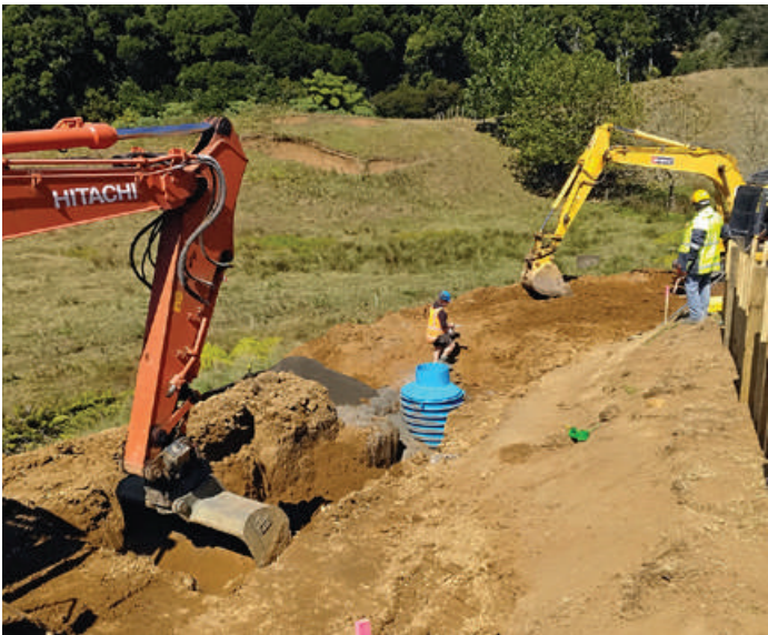
Patterson Road - Sutherland Sewer
