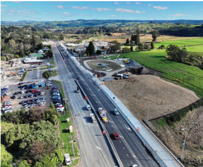
Tauriko West Enabling Works
