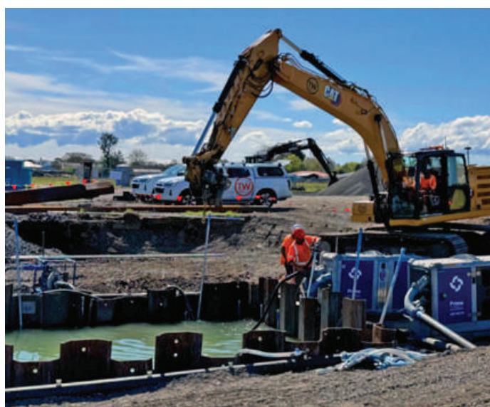
Hastings Developments - Wastewater Upgrades
