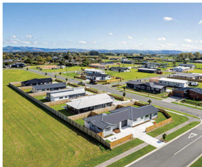
Taruheru Catchment - Oakview Housing Development
