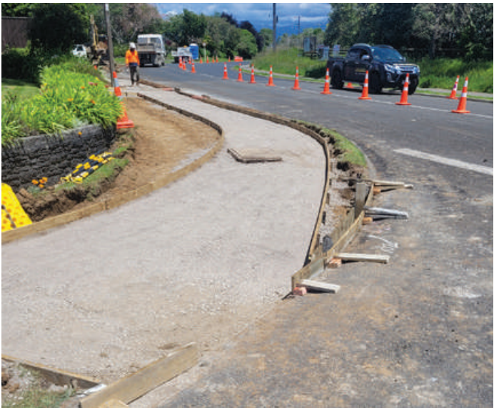
Patterson Road - Frankley Road Shared Pathway
