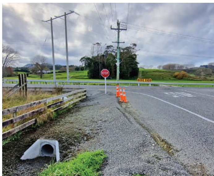
Taruheru Catchment - Hansen Road New Culvert
