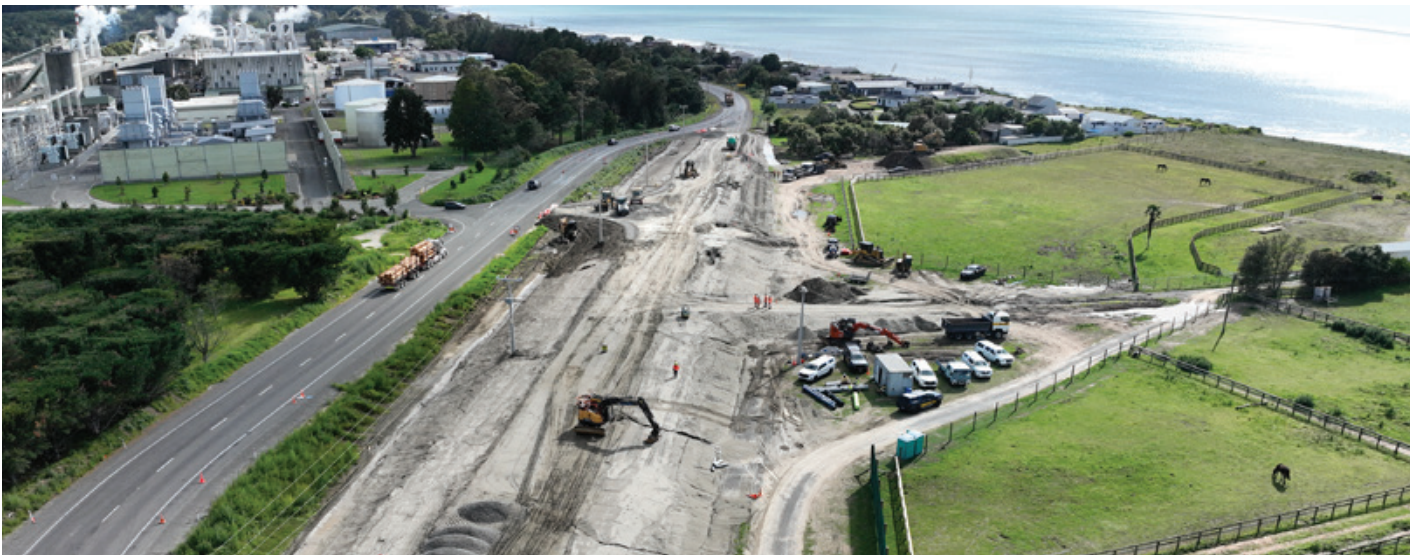
Whirinaki Flood Mitigation, Hawke's Bay Regional Council
