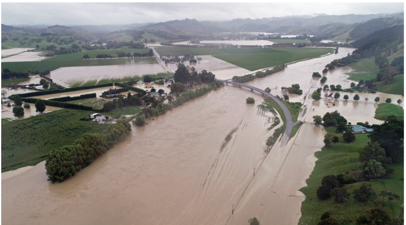
Kaitaratahi Bridge during Cyclone Gabrielle
