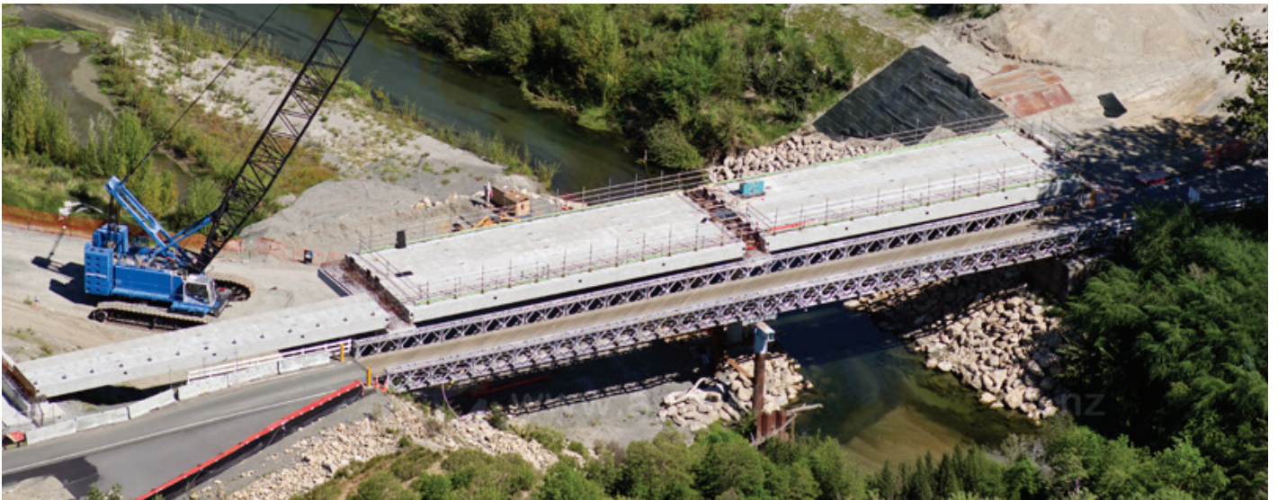
Rissington Bridge, Hastings District Council
