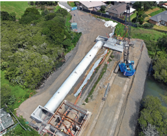
Harania Creek Flood Resilience Project, Auckland Council
