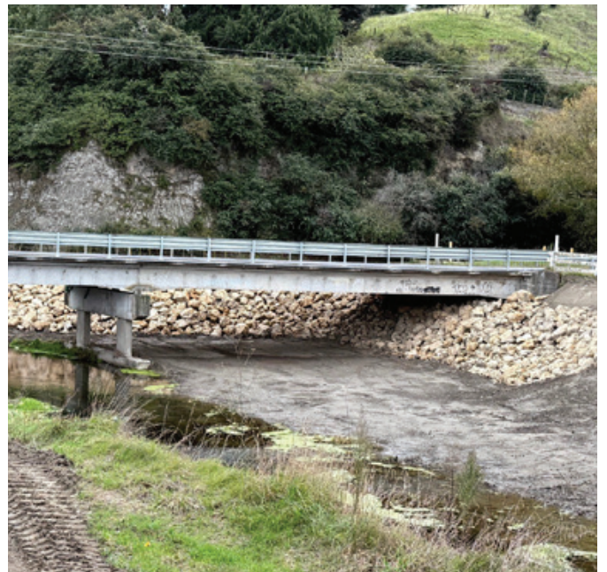
Okawa Stream rock armour works under Taihape Bridge
