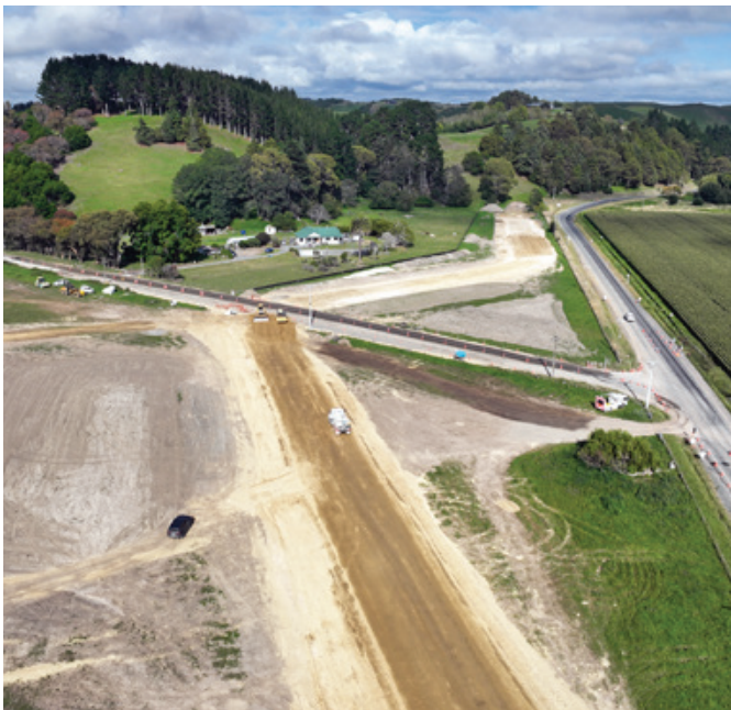
Ōhiti Road Stopbank Construction
