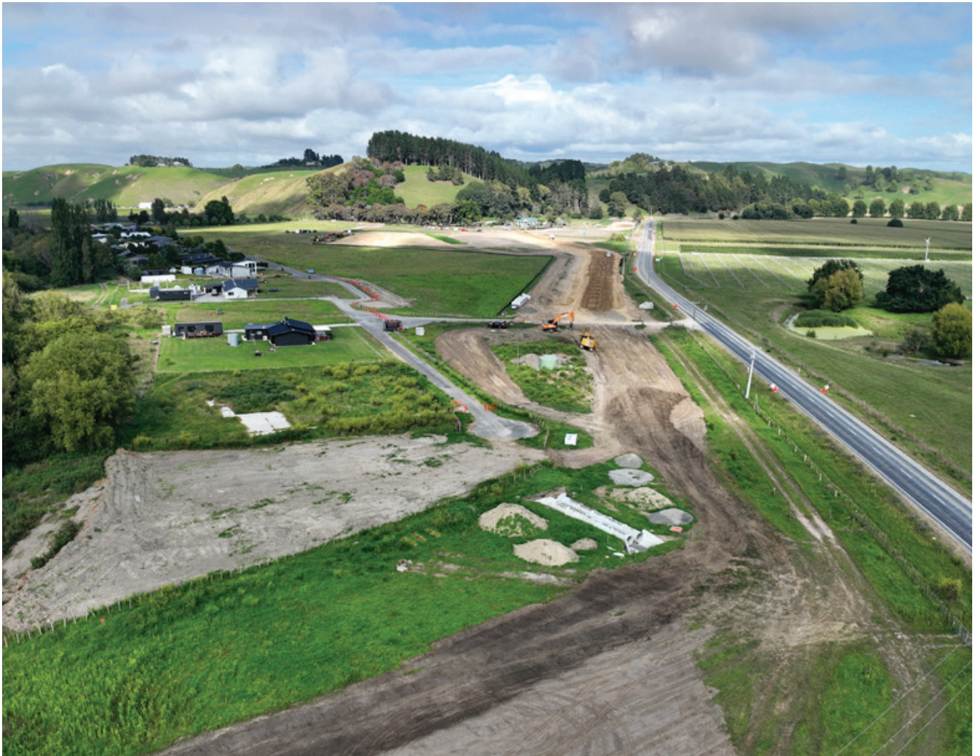
Ōhiti Road Stopbank Construction
