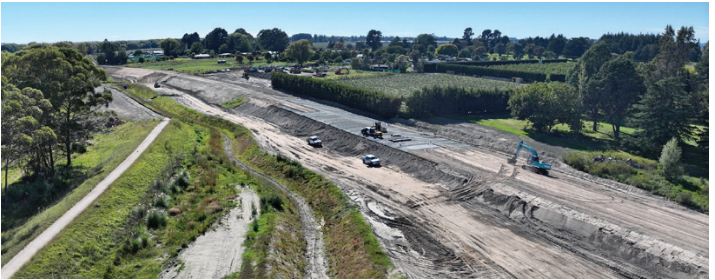
Waiohiki Flood Mitigation, Hawke's Bay Regional Council
