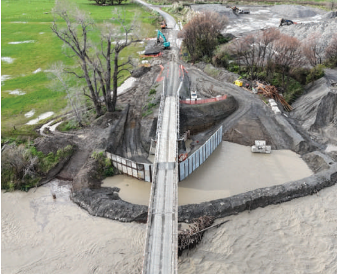
Makarika Bridge, Gisborne District Council
