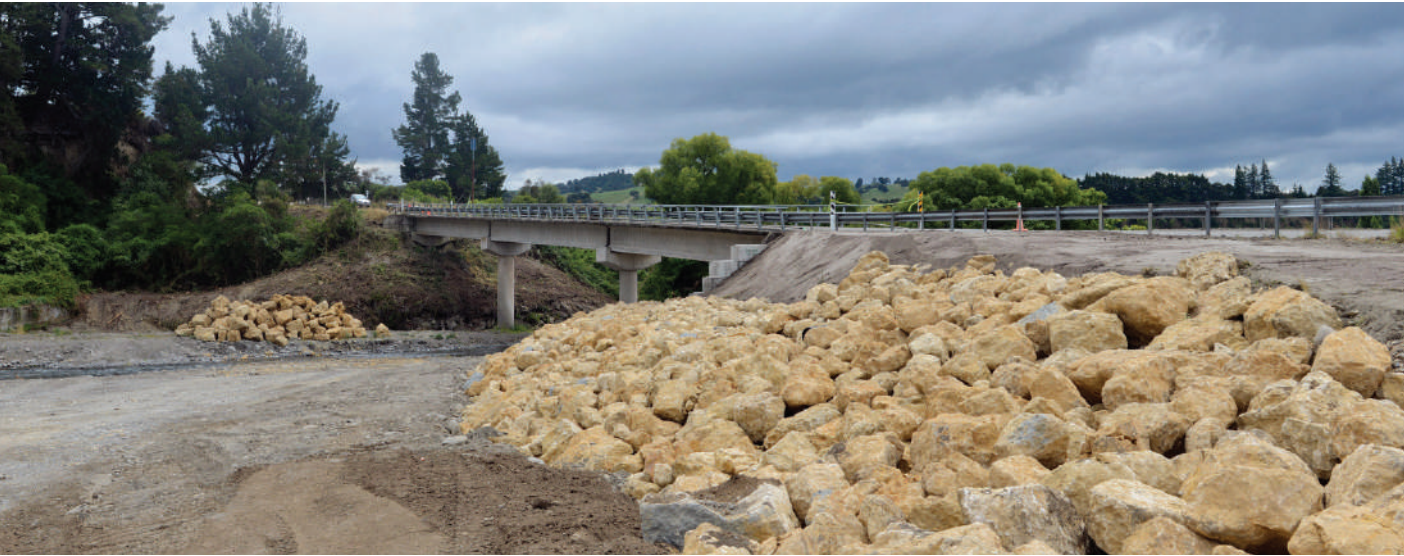
Central Hawke's Bay District Council, Fletchers Crossing Bridge rebuild
