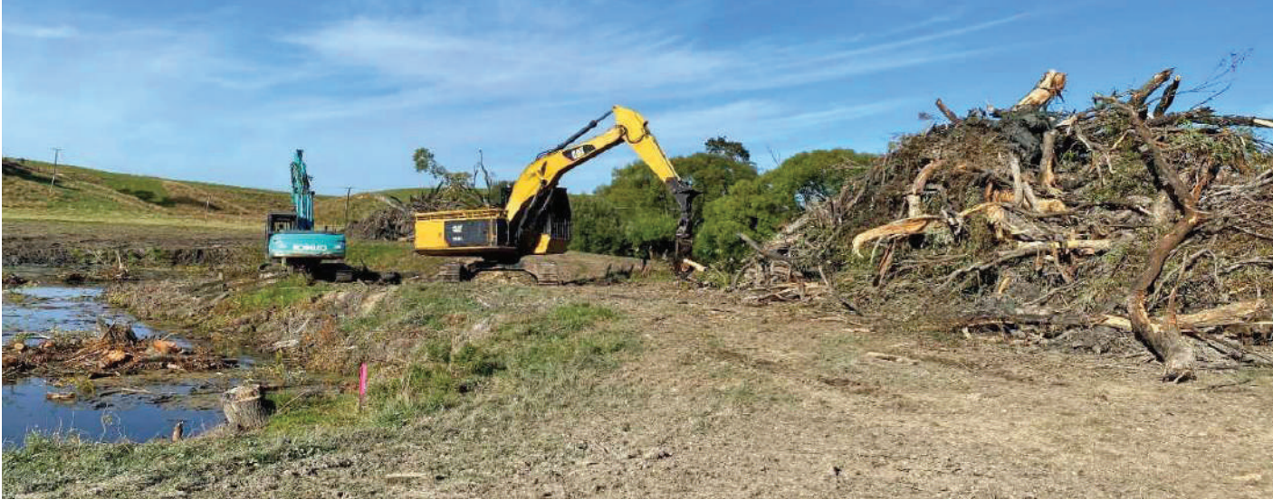
Greater Wellington Regional Council, Whangaehu River blockage removal
