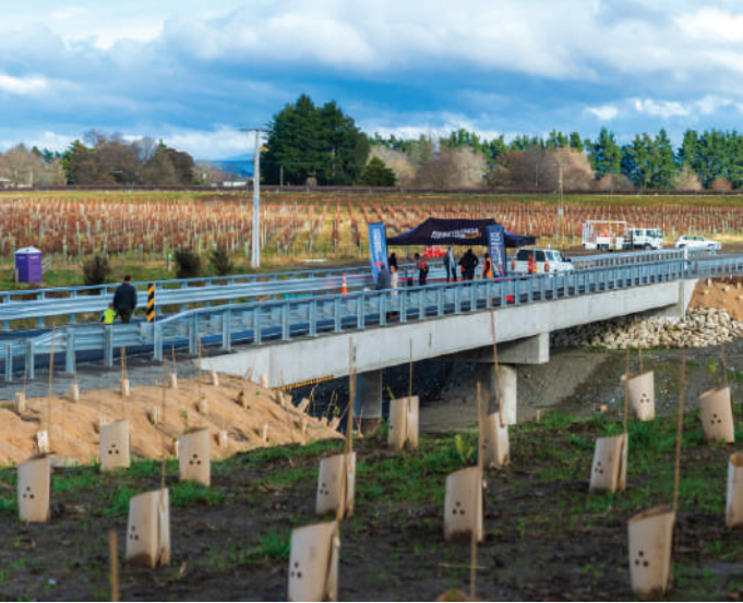
Matapiro Bridge, Hastings District Council
