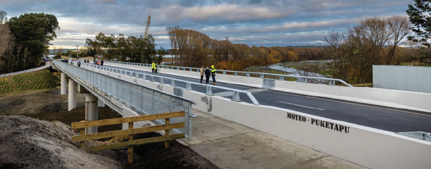
Moteo-Puketapu Bridge, Hastings District Council
