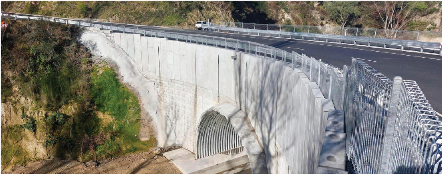
Hastings District Council, Kereru Gorge Culvert
