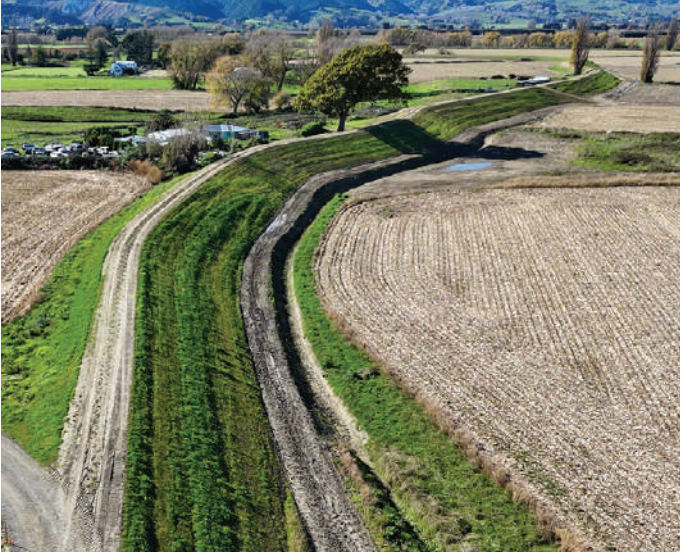
Waipaoa Stopbanks, Gisborne District Council
