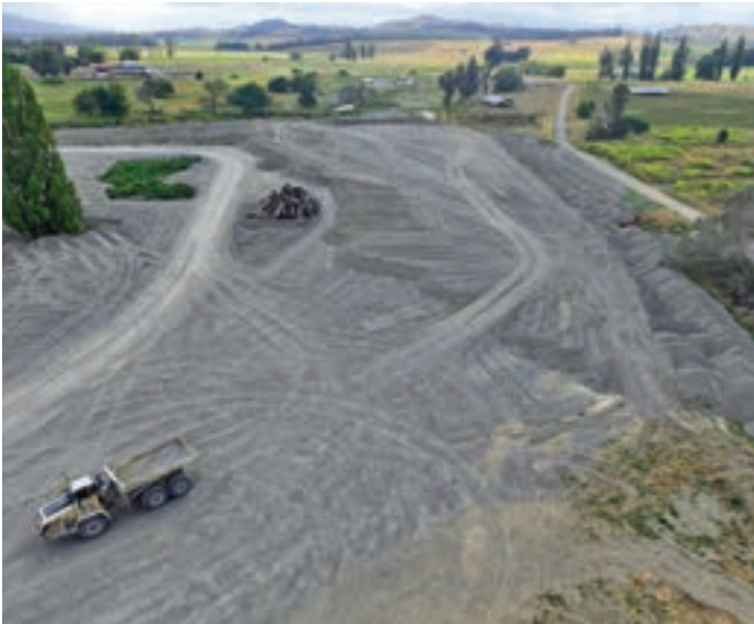
Upper Tukituki Flood Control Scheme
