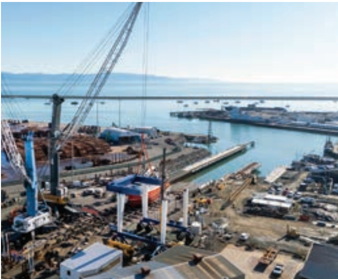
AIMEX Nelson Port Slipway
