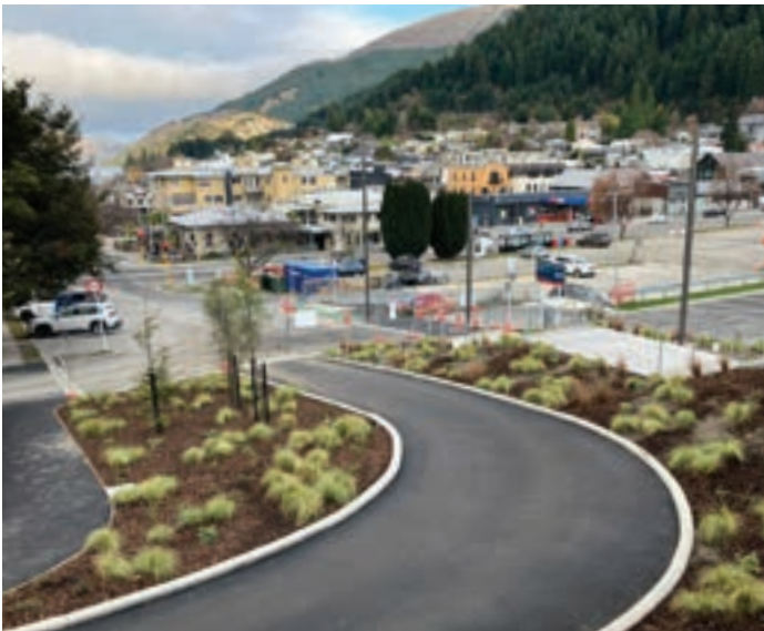
Queenstown Arterials - Stage 1
