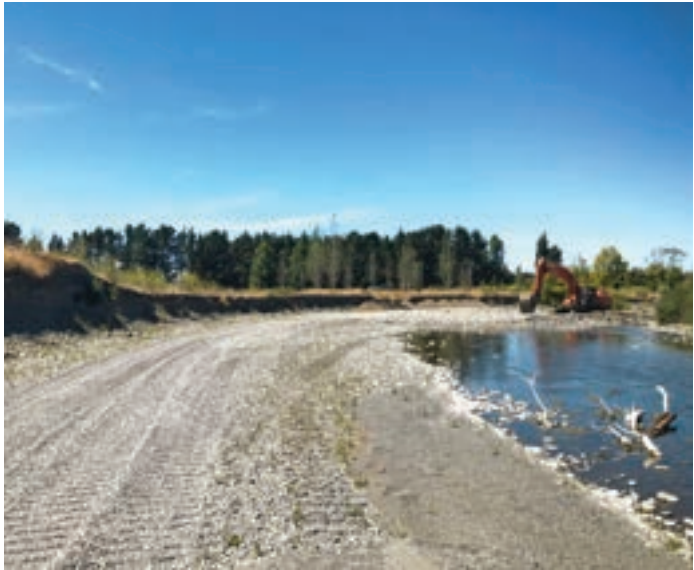
Upper Tukituki Flood Control Scheme
