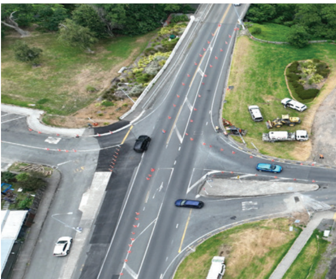
Galbraith Street - Ngāruawāhia - Old Taupiri Rd - Great South Rd Intersection
