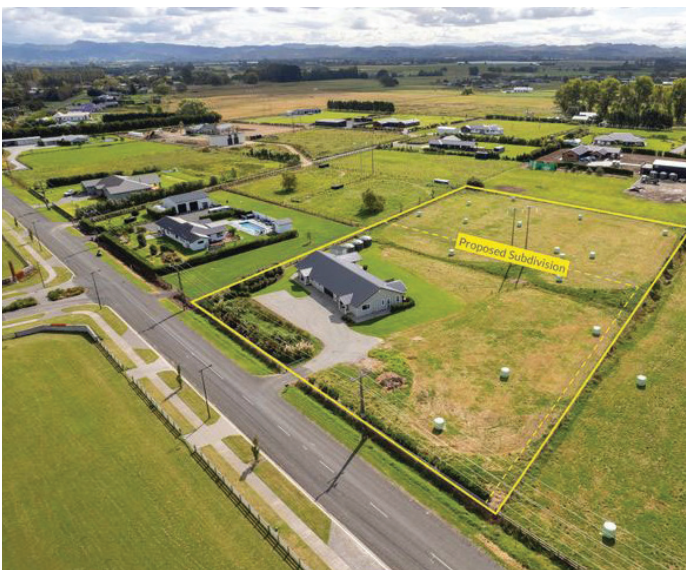
Taruheru Catchment - Hansen Road upgrade
