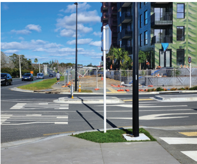
Carrington Residential Development - Carrington Road Enabling
