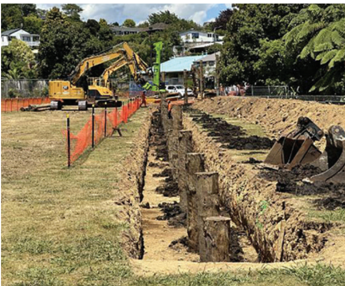
Patterson Road - Sutherland Sewer
