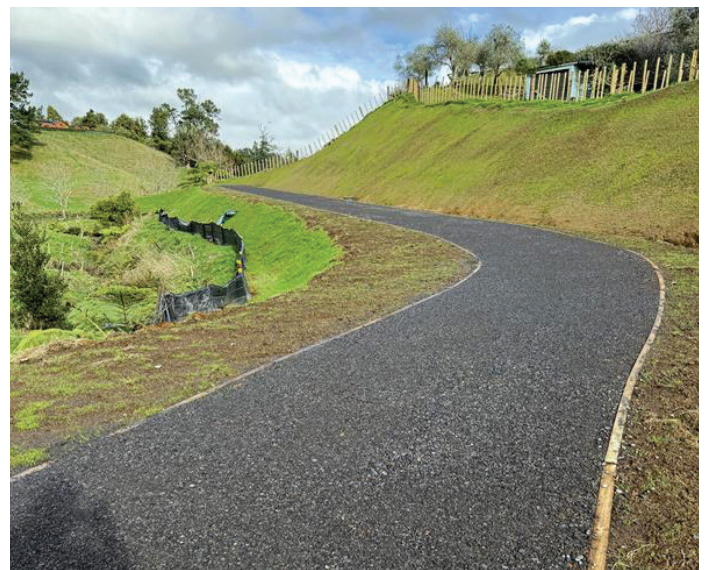
Patterson Road - Sutherland Cycleway & Walkway
