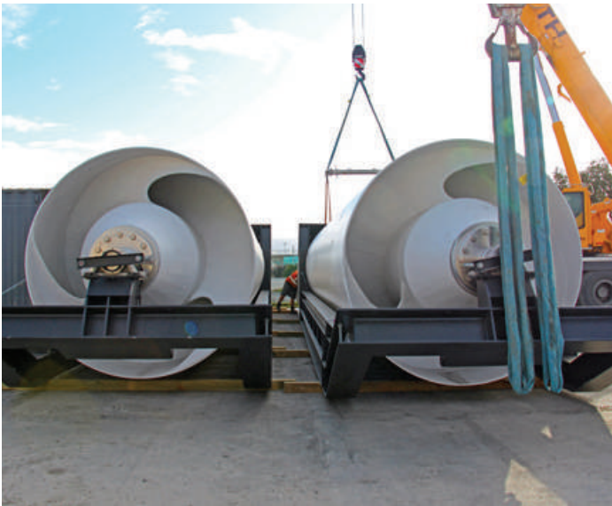
Stead Street Pumpstation
