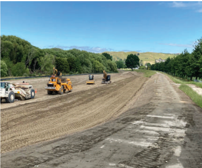
Heretaunga Plains Flood Control Protection
