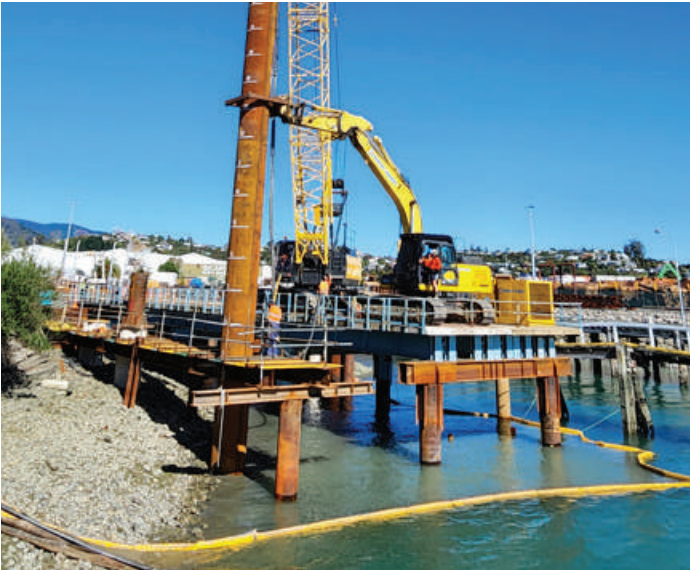
AIMEX Nelson Port Slipway
