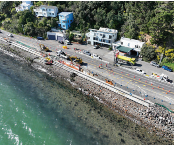
Eastern Bays Shared Path
