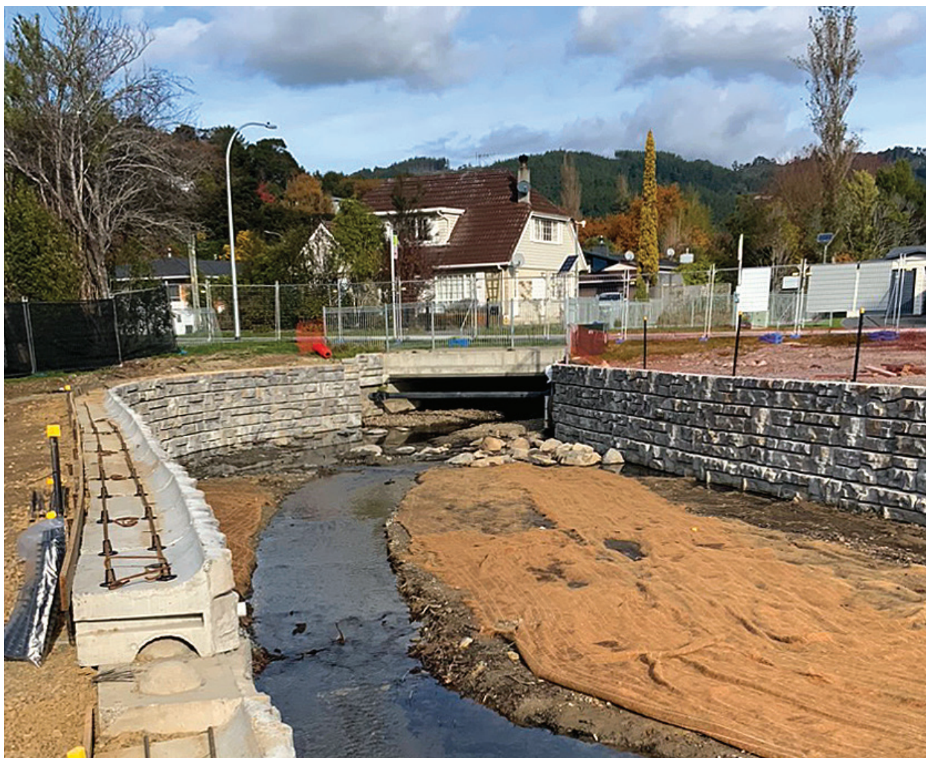
Pinehaven Stream improvements Phase 2, Upper Hutt City Council (completed 1 March 2024)
