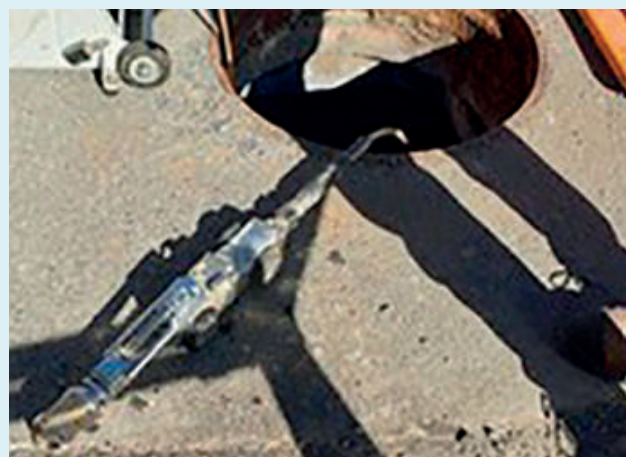
Wellington Wastewater CCTV set up
