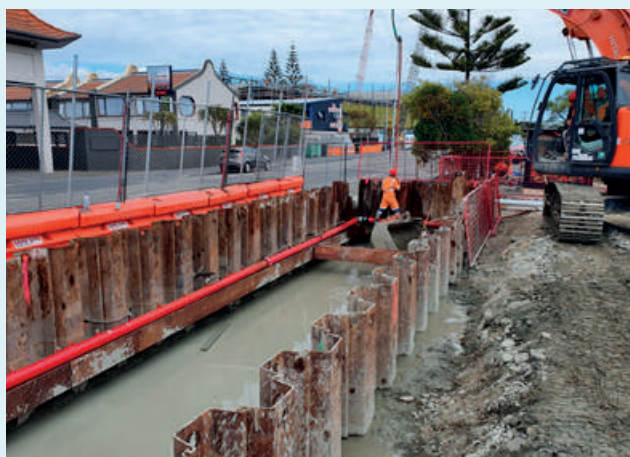
Wastewater storage tank upgrade, Nelson City Council
