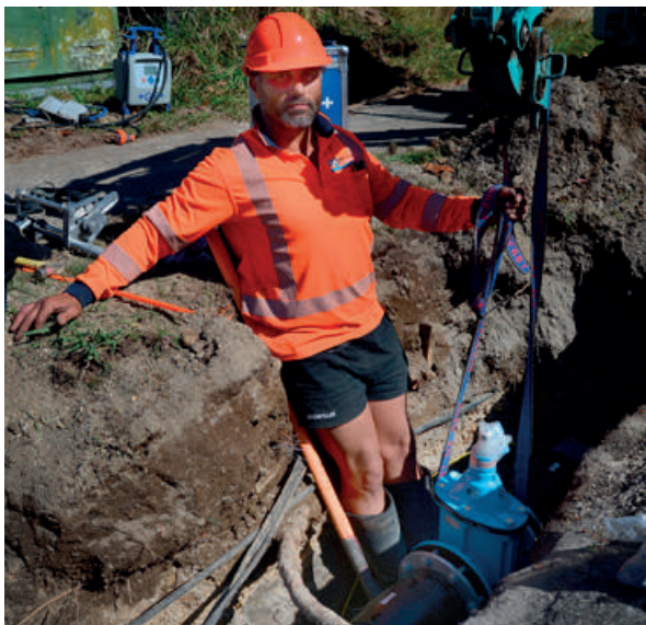
Valve installation for water network renewals.
