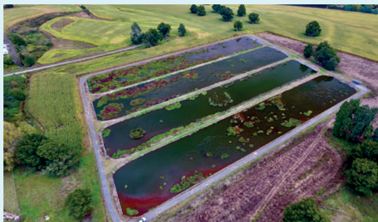
Hikumutu Waste Water Treatment Plant upgrade, Ruapehu D.C.
