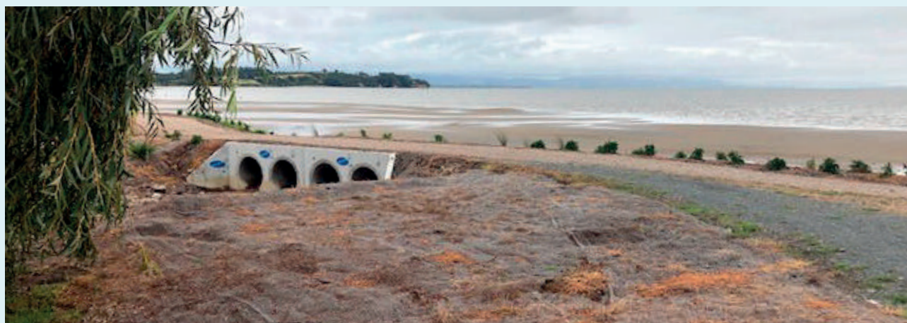
Omokoroa Storm Water Bund
