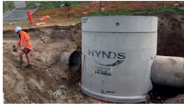
Installation of the Defender Unit as part of the Hawai Street Stormwater project.
