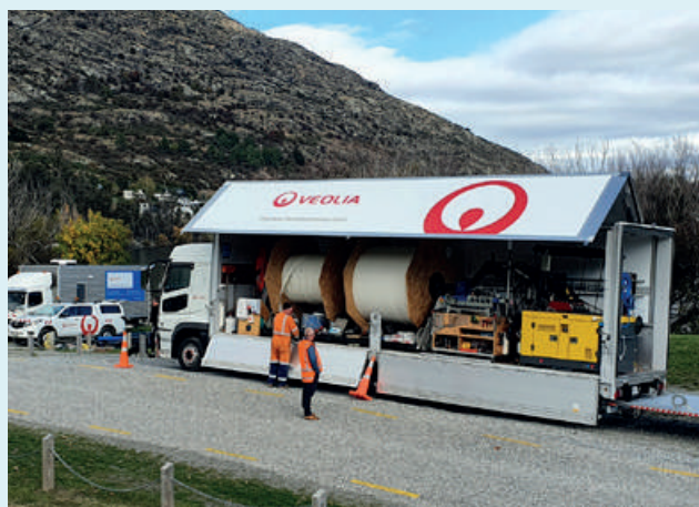
QLDC - Lining of Wastewater Mains
