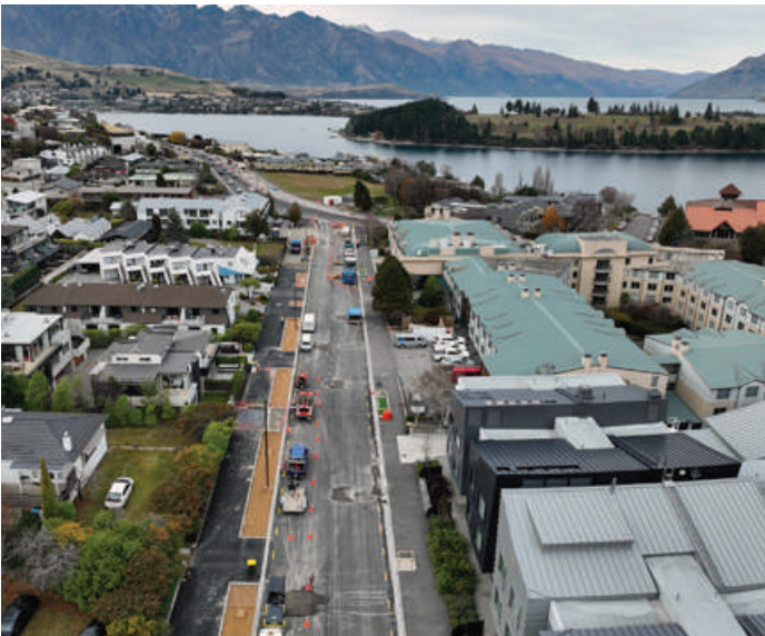
Queenstown Arterials - Stage 1
