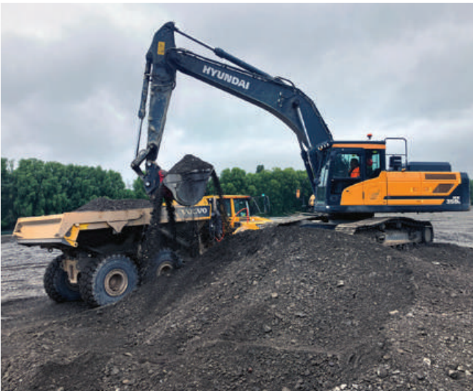
Upper Tukituki Flood Control Scheme
