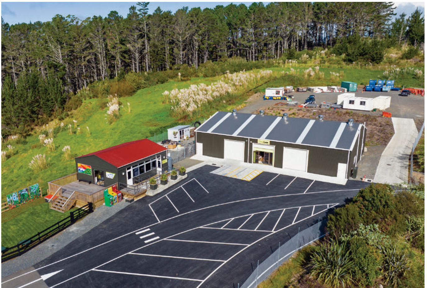
Warkworth Community Recycling Centre, Auckland Resource Recovery Network
