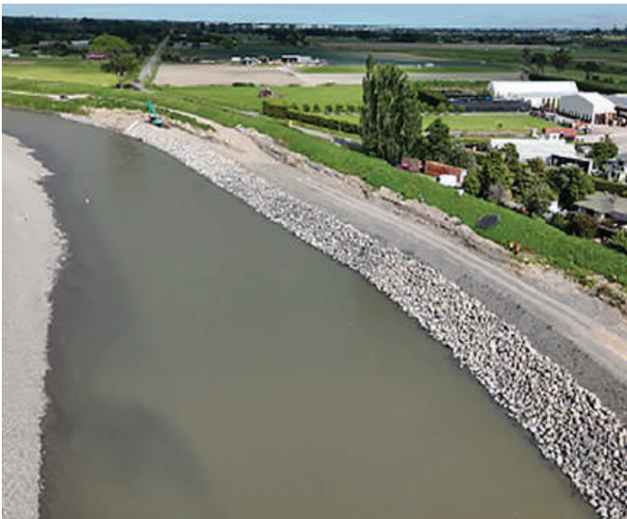
Lower Manawatu Flood Protection Resilience
