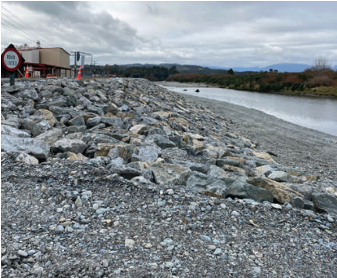
Hokitika Beach Coastal Protection Project
