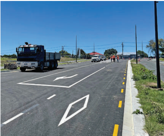
Unitec Housing Development
