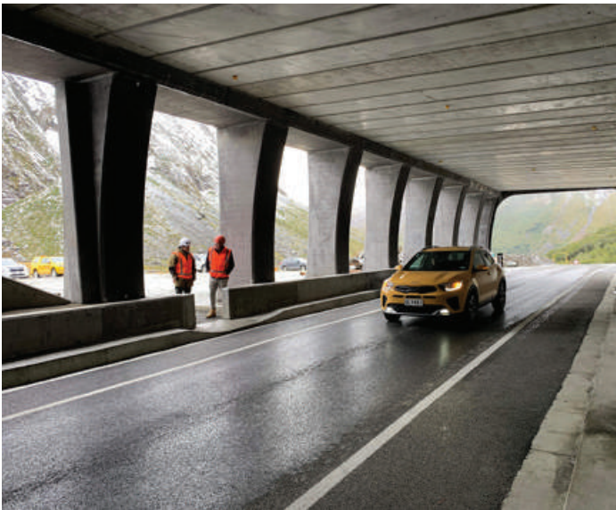
SH94 Homer Tunnel
