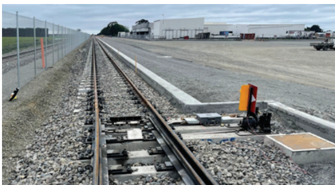
Ashburton District Council - Fairfield Freight Hub KiwiRail interchange
