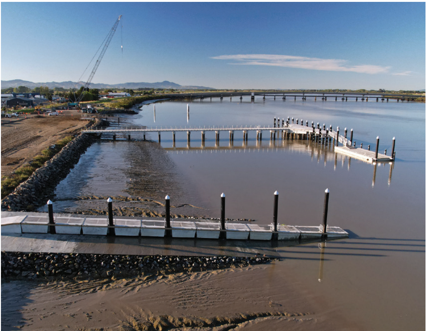
Thames-Coromandel District Council - installation of commercial wharf fender piles
