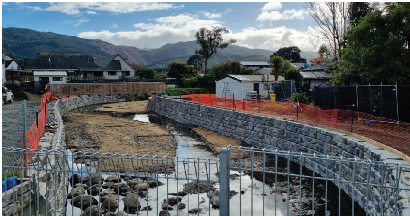
Pinehaven Stream improvements Phase 2, Upper Hutt City Council (completed 1 March 2024)
