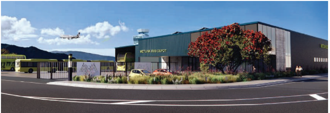
Electric Bus Depot, Lyall Bay, Wellington, Greater Wellington Regional Council (completed June 2024)
